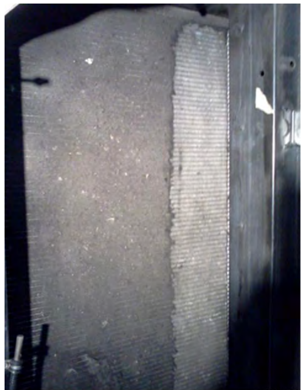
Figure 244: Coil after Wiping Right Hand Side with Cloth
